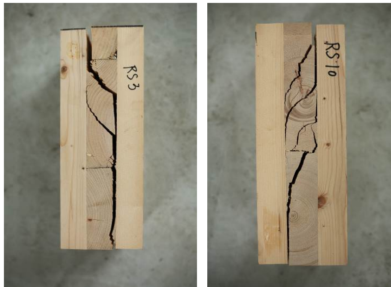
Figure 11: Rolling shear failure in compression shear tests
